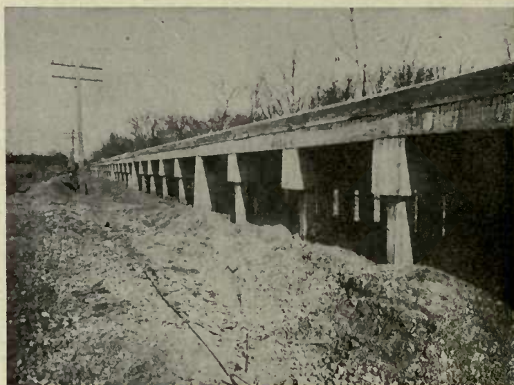
FIG. 167.—FIRST CONCRETE TRESTLE. CHICAGO, BURLINGTON & QUINCY RAILWAY.
