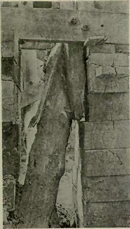
FIG. 18d.—PILE TELESCOPED IN DRIVING.
