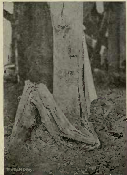
FIG. 18g.—PILE BUCKLED, SLIVERED, AND BENT IN TWO DIRECTIONS.
