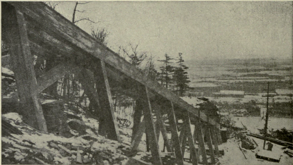
PLATE LXXIV.—CONCRETE TRESTLE, OTIS ELEVATING RAILWAY.
