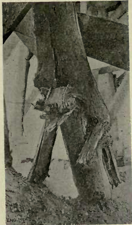
FIG. 18e.—PILE TELESCOPED IN DRIVING.
