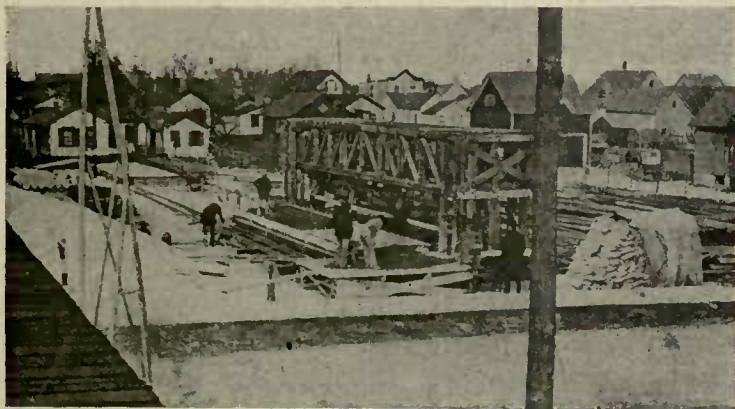
FIG. 172.—GENERAL VIEW OF PLANT FOR CONCRETE PILES.
