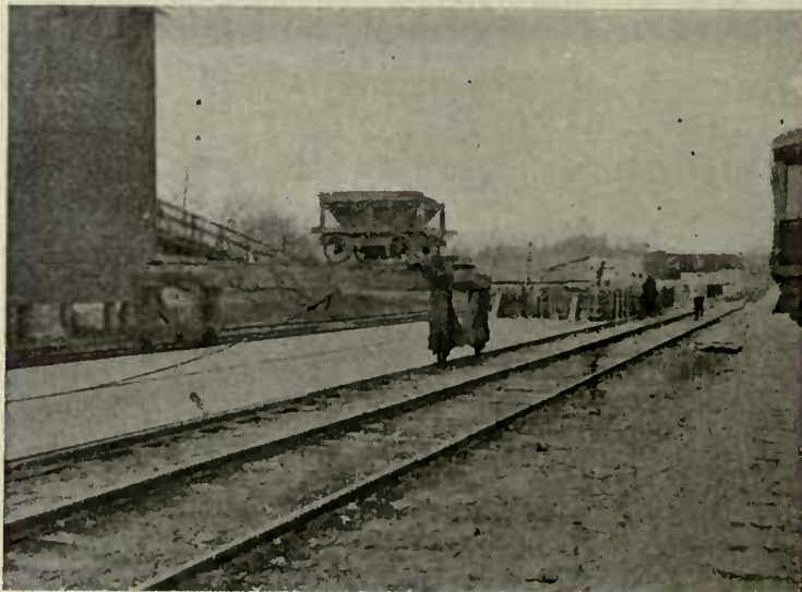
FIG. 177.—PLANT FOR FLOOR SLABS.
